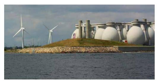
**Figure 1.** MWRA's facilities: 98% of the plants heating needs and 22% of the plant's electricity needs are created in-house through the process
